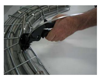
3. Squeeze the handle to tighten tie to the desired tension.
