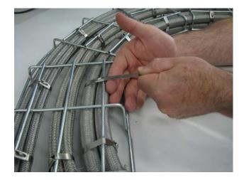
1. Loop cable tie around bundle. Insert the tail into the buckle and pull tight by hand.
