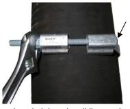
Bolt must be flush with retainer surface
